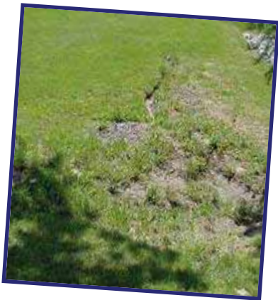
Failing septic field
