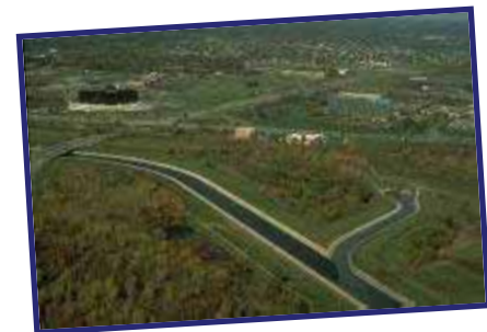
Concrete channel in the Main 3-4 Subwatershed
