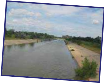
Concrete channel in Dearborn
