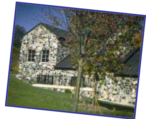
Linden Park CSO in Birmingham
