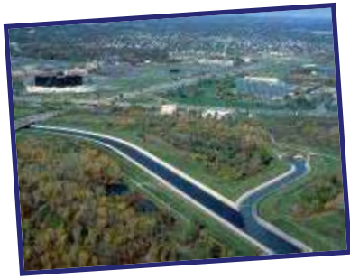
Channelized area of the Rouge River in Dearborn
