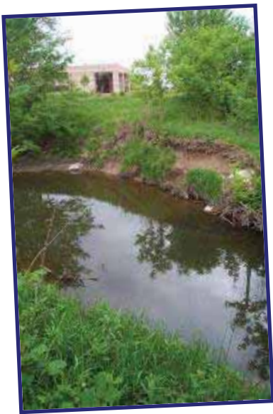
Eroded streambank in Tonquish Creek
