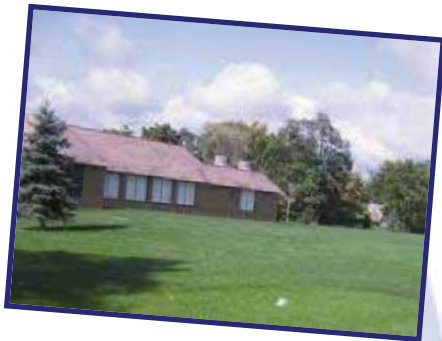
CSO basin in Redford
