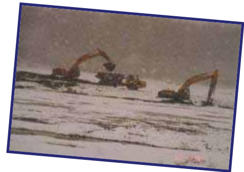
Sediment removal at Newburgh Lake in Livonia
