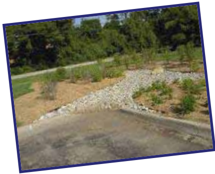
Rain garden in the City of Troy
