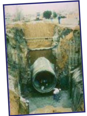
Garden City sewer separation project
